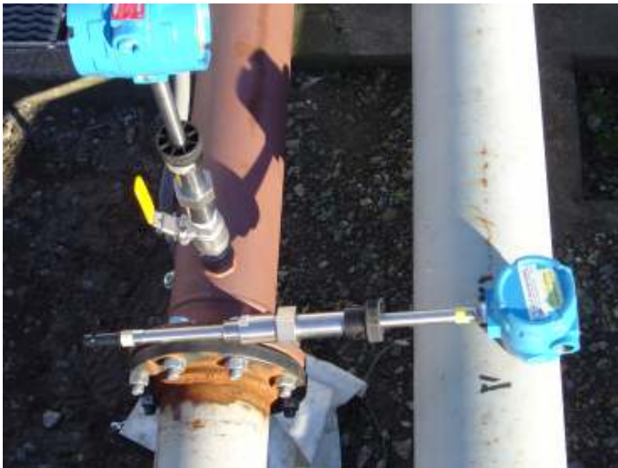
Figure 3 D-2 JF-1A On-Line Fuel Sensor With Retractable Mount
